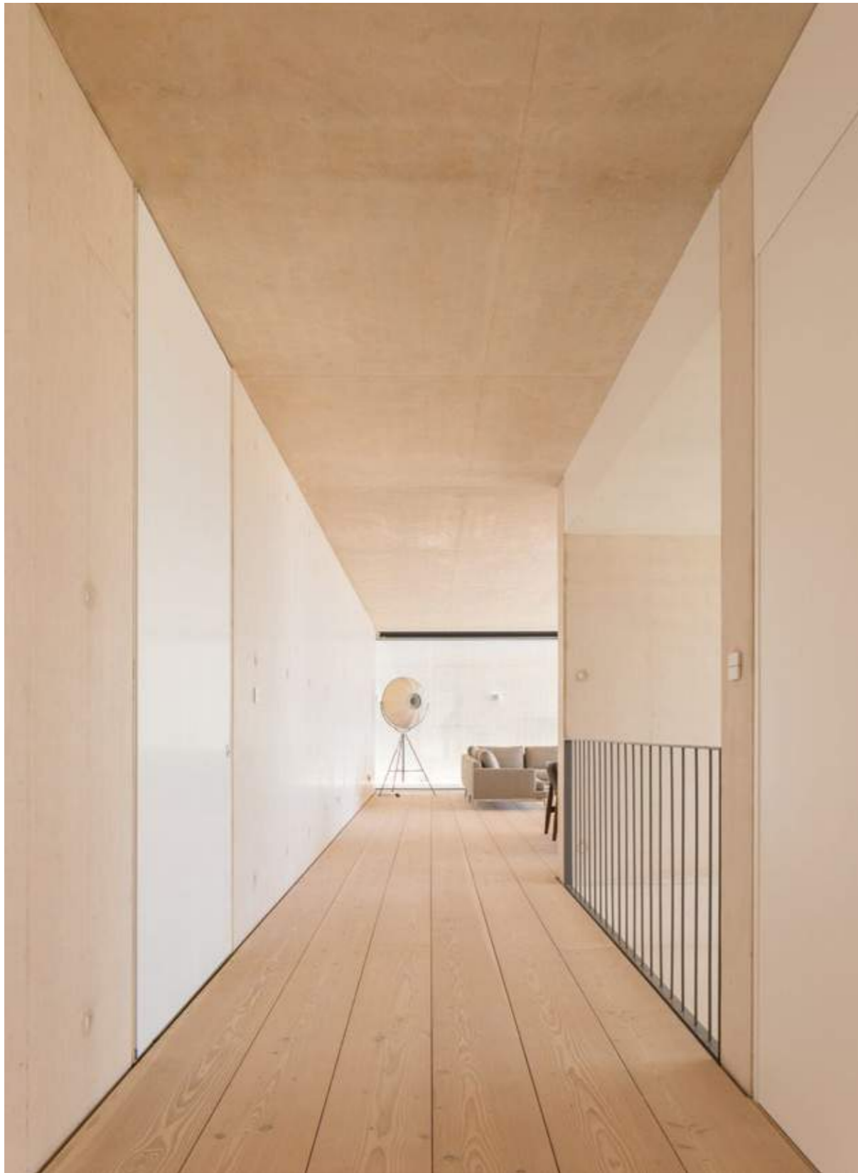
pur natur Floorboards Douglas Select 28×300mm Full lengths up to 15m white lye + white soap
